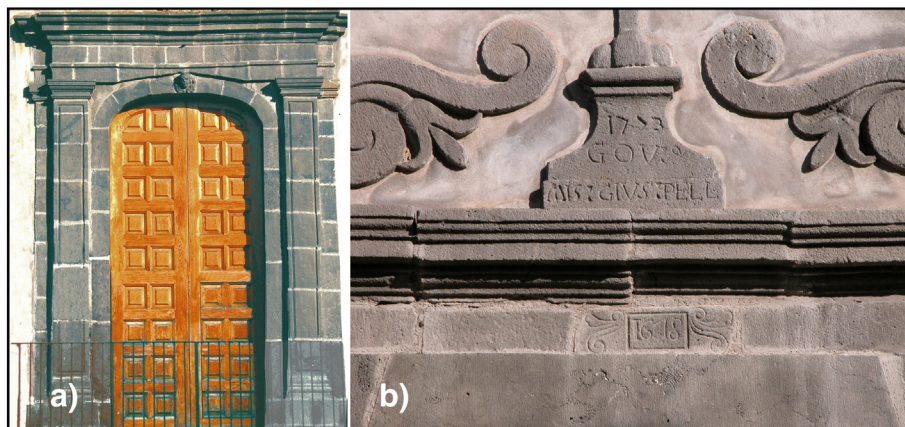
Fig. 10. Belpasso. a) The portal of the original church of St. Antony which was removed from Fencia Moncada following the 1693 earthquakes and was re-mounted in the church that was rebuilt in the new settlement. b) Details of a lintel which commemorate the building of the old church in 1678 (bottom) and new church in 1773 (top). Photographs by R. Azzaro.
